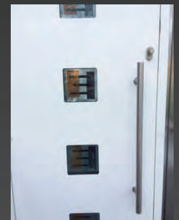
Internal view of door
